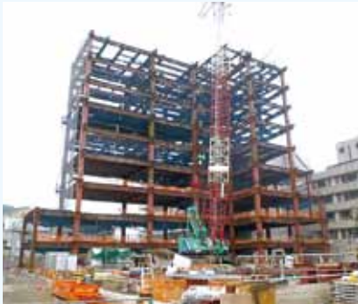
鉄骨建方① (8/9)
